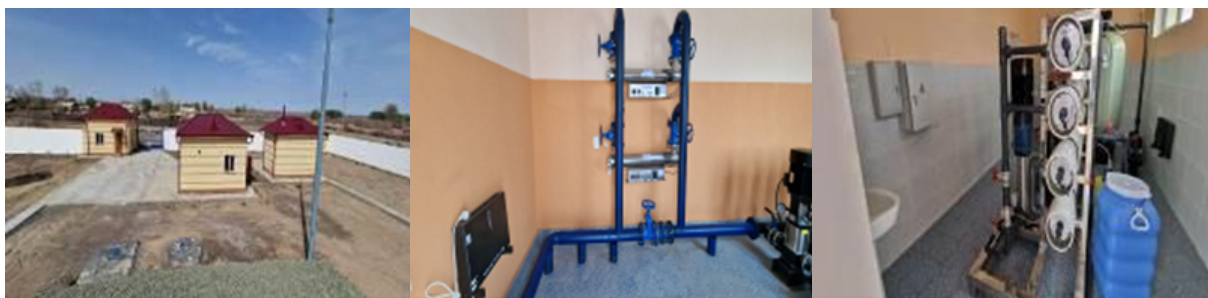
Photos 56, 57, 58: Water project on access to clean drinking water in Taza jol VCC of Chimbay district.
